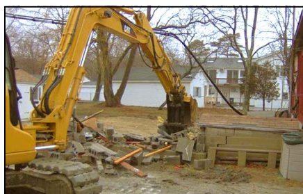
RAZING THE CINDER BLOCK OIL FURNACE BUILDING
