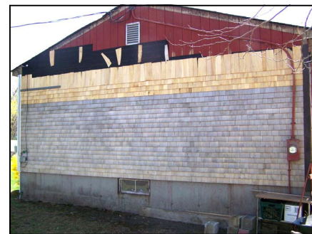
MORE SHINGLES ARE BEING ADDED EACH SUNDAY
