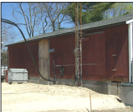
REGRADED - PHASE 2 BASE OF THE TOWER NEEDS TO BE CAREFULLY FILLED
