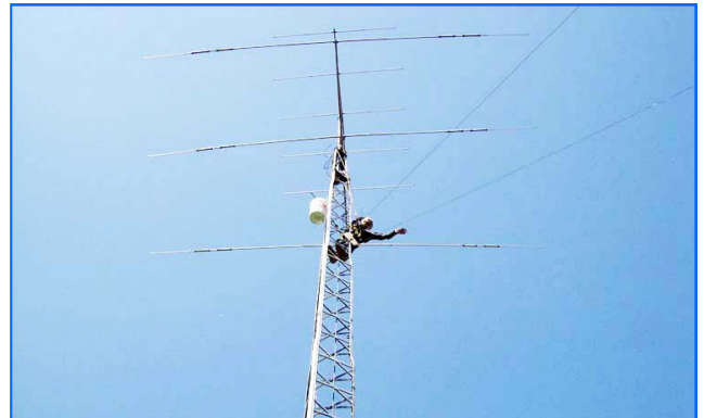
JOHN-WA1LSH DOING TOWER WORK. ABOVE THE TRI-BANDER IS A 5-EL 6-M YAGI.
