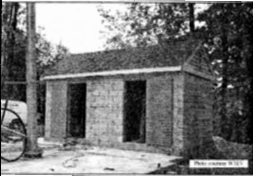
TRANSMITTER BUILDING AT TOWER SITE
