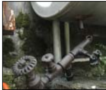
BROKEN ELBOW
