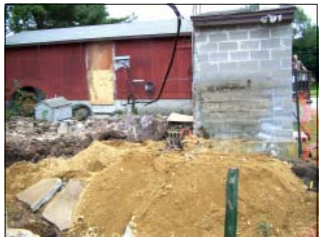
MORE BACK FILL TO STABILIZE THE BUILDING
