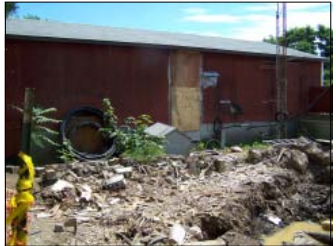
NORTH SIDE OF THE CLUB HOUSE
