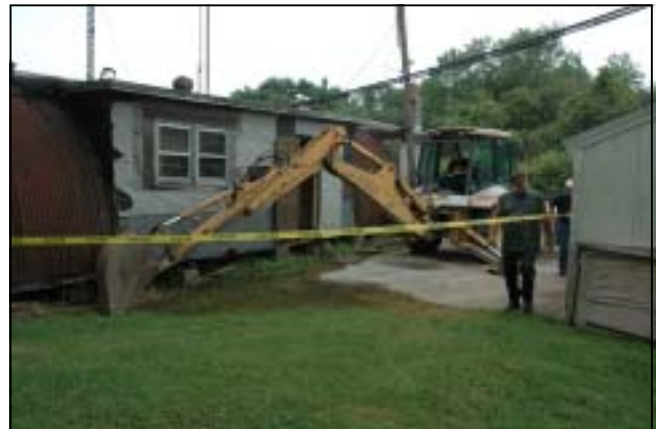
DIGGING THE FIRST TRENCH
