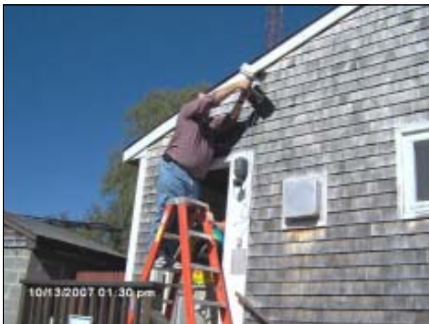
DAVE, W1DJG DOING THE INSTALL
