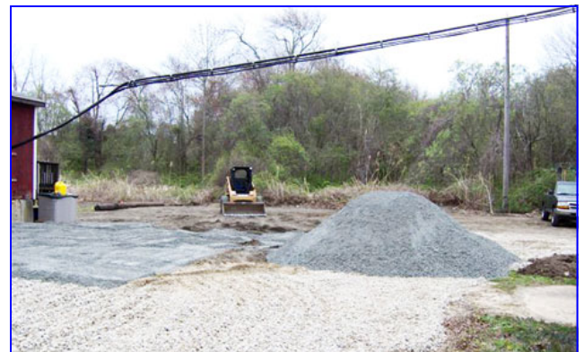
START OF REGRADING ON THE DRIVEWAY
