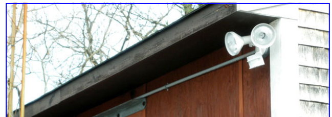
THE NEWLY INSTALLED MOTION-SENSOR LIGHT
