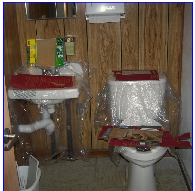
NEW FIXTURES HAVE BEEN INSTALLED — NOT READY FOR PRIME TIME YET —
